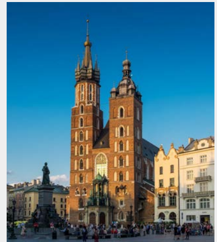
St. Mary's Church, Cracow
